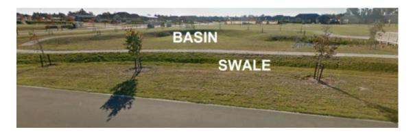
Swales are seen as a low lying channel next to a road or street. These streets do not have curbs allowing the rainwater to flow directly into the swale and down towards a stormwater basin.
